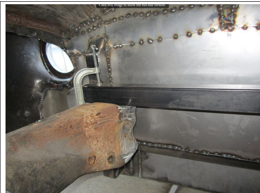
The grill area is blocked off and I have front body mounts near there. A majority of the work on this car is where it will never be seen.
