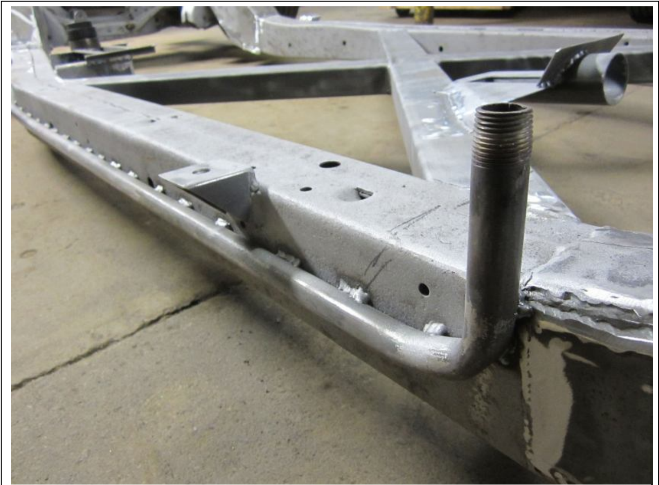
My air lines are 1/2 inch black pipe welded directly to the frame.
