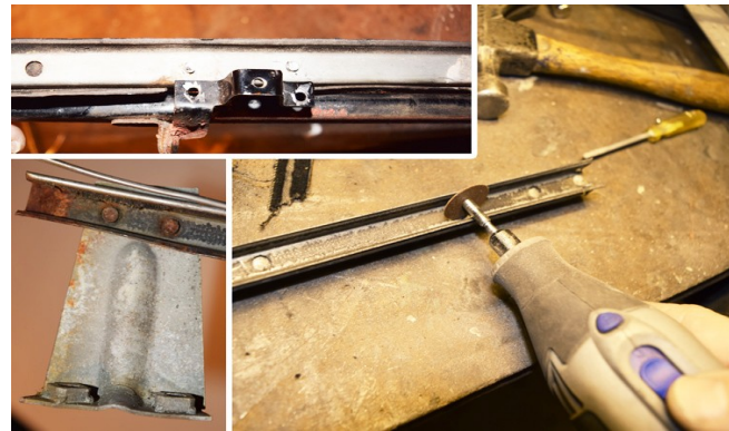
Figure 2. Grinding off rivet heads.
