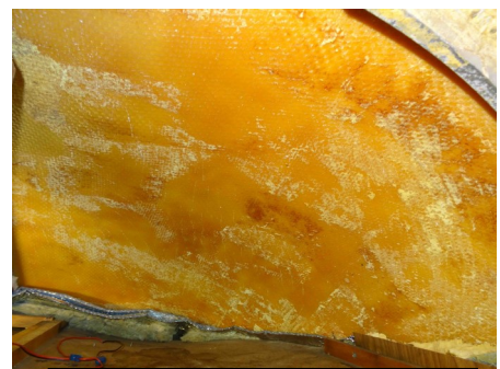
Driver's side under the fiberglass corner with the foam removed
