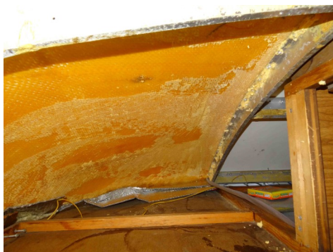
Passenger's side under the fiberglass corner with the foam removed
