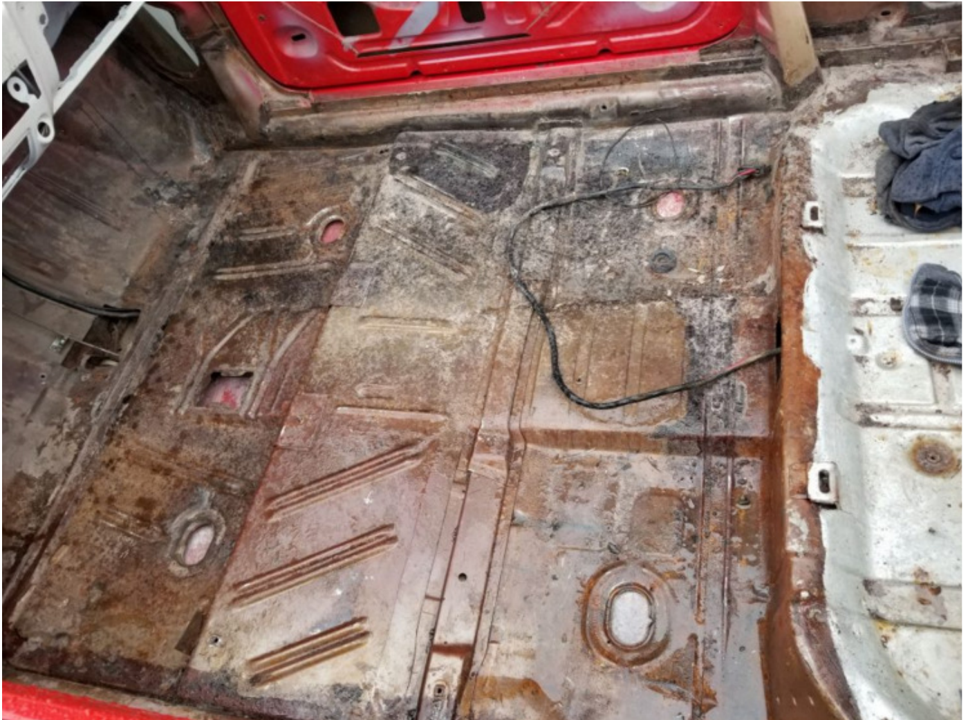
The floor, on the other hand, is solid and not corroded.
