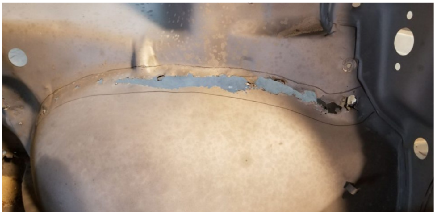
The right front wheel well, inside the luggage compartment showing what needs to be cut away and replaced.
