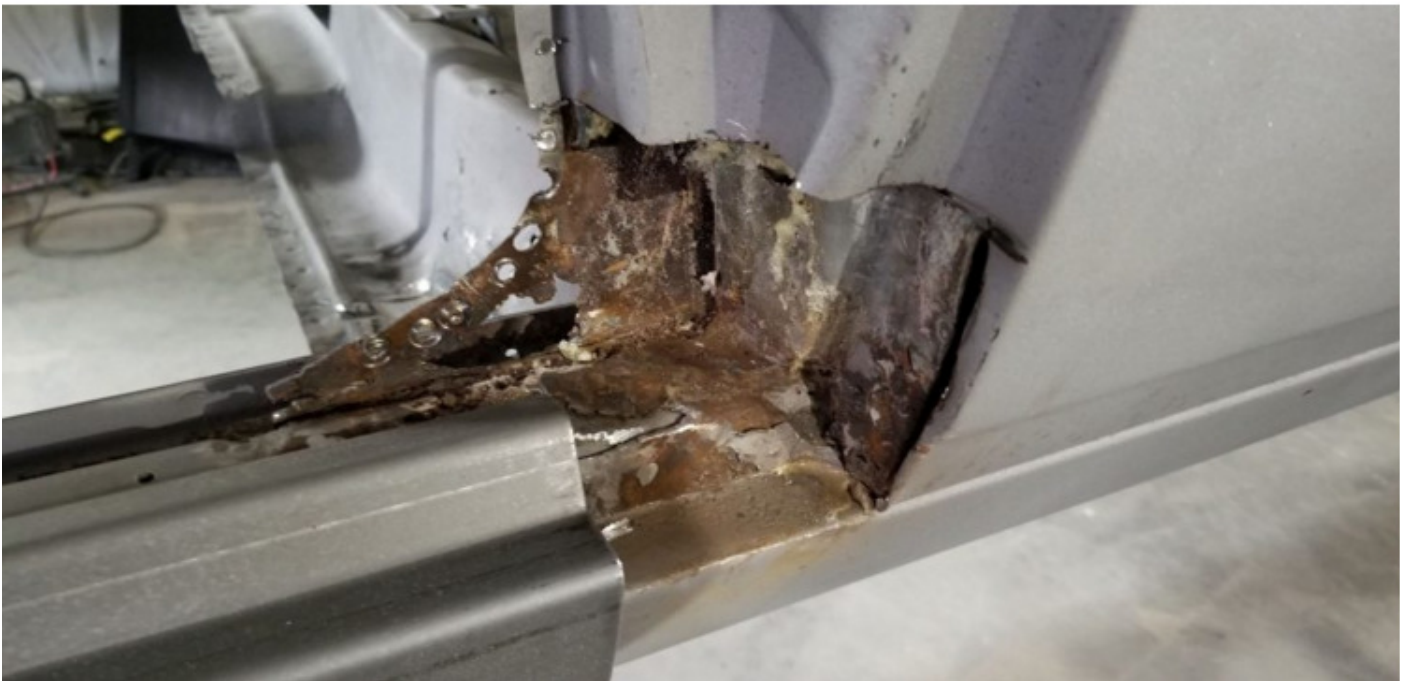
The same area, with much of the corrosion cut out.
