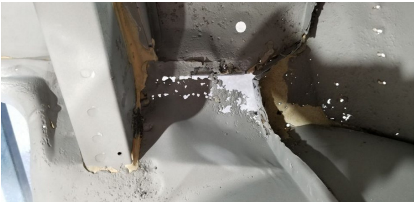
Right rear, also behind the engine. Both areas will require patch panels.
