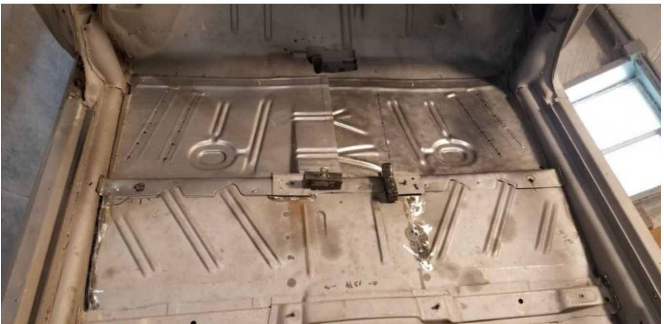
New front floor pans are welded in
