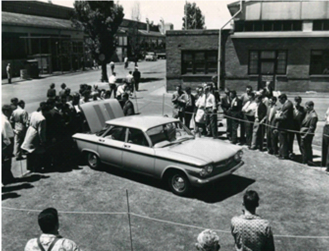
Photo 1. The location is the General Motors Holden (GMH) Fisherman's Bend assembly plant. The photo was likely taken between late 1959 to early 1960.
