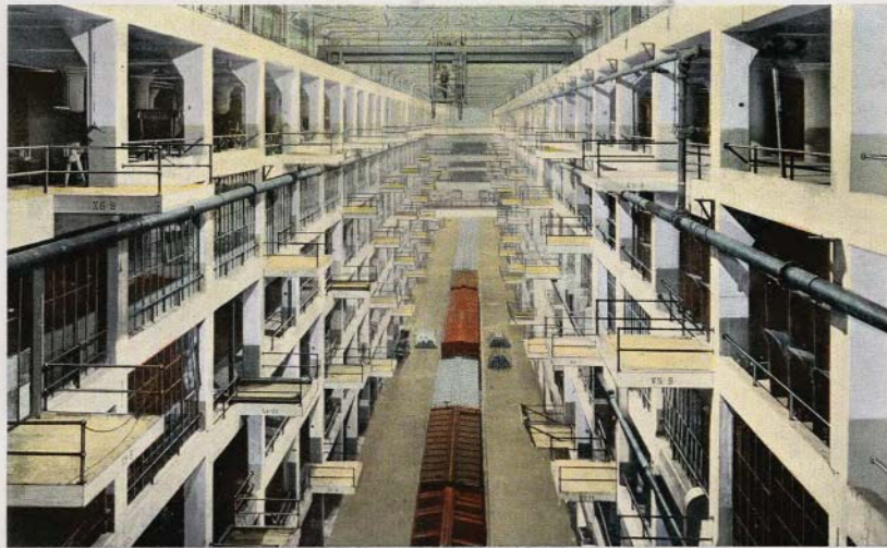
CRANEWAY IN NEW 6-STORY BUILDING, SHOWING LOADING PLATFORMS.
