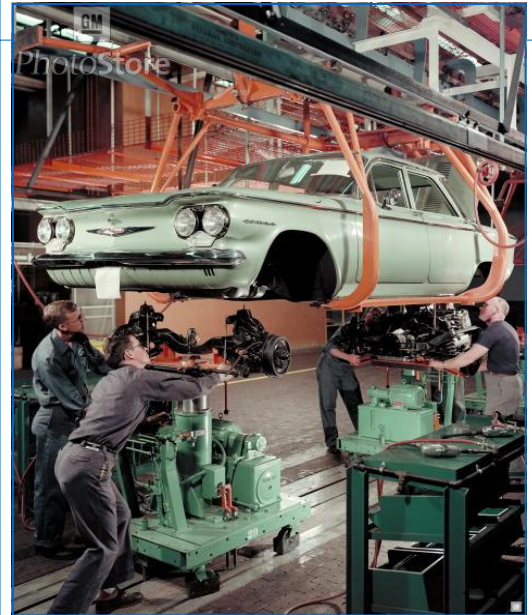
1960 Corvair on Assembly Line
